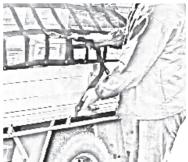
5) Pull the cam buckle straps tight to secure the load snugly.
